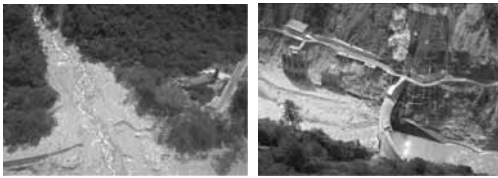
Figure 3. (a) Destructive debris flow occurred. (b) Hydro-power facilities damaged by debris flow during the Mindulle typhoon.
